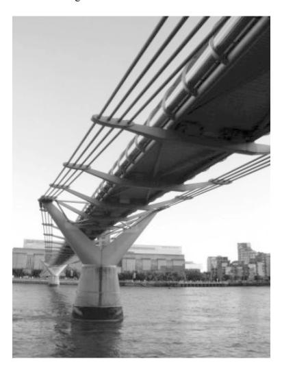
To solve the problem the engineers decided to use damping mechanisms – giant shock absorbers to limit the bridge's response to external forces. They decided to use two systems: viscous dampers, similar to car shock absorbers, and tuned mass dampers. A tuned mass damper is a large mass stiffened by springs.
